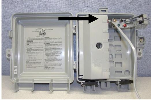
Figure 3: Plug telephone cord into the jack.
